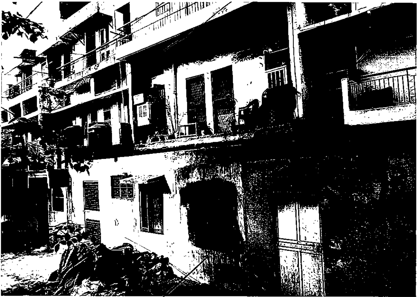
REAR COURTYARDS COVERED AT A LOWER LEVEL ALMOST 2'-6" - 3'-0" BELOW BY ALMOST ALL GROUND FLOOR OWNERS
